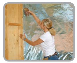
CHANNELS MOISTURE VAPOR AND ALLOWS FOR BREATHEABILITY - when vapor enters the attic from the living space, THERMO REFLECT ATTIC NT helps diffuse the vapor through its breathable membrane.
