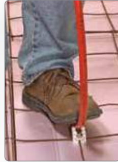
Protective plastic-to-plastic PEX connections
