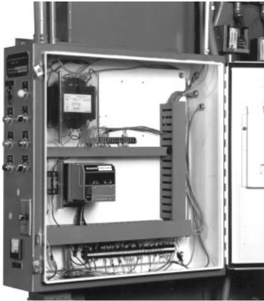
Fig. 7. Electrical panel installation.
