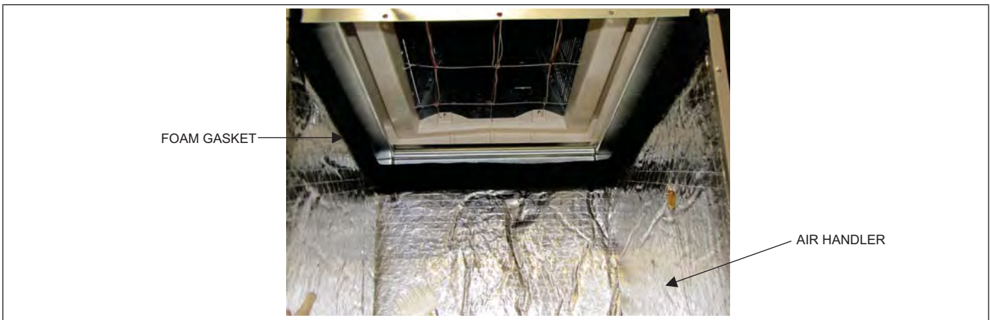
FIGURE 4: Gasket Location
