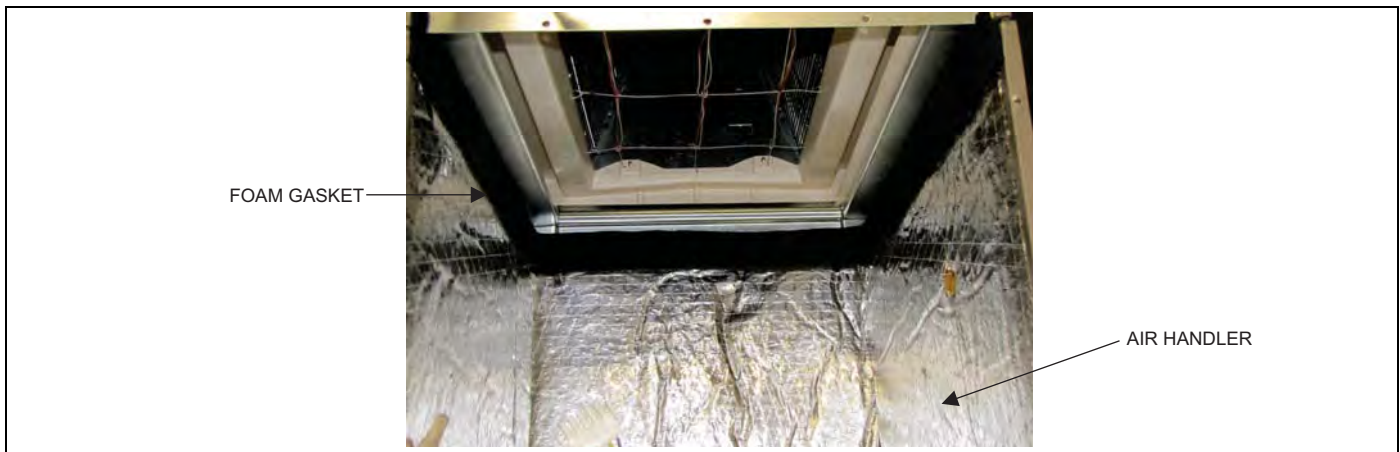
FIGURE 4: Gasket Location
