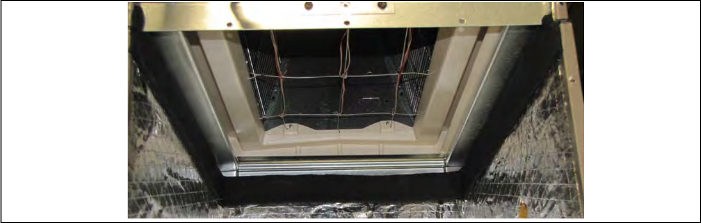
FIGURE 3: Gasket Location
